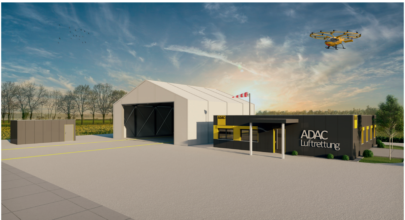
Figure 9.1: Container station with lightweight hangar
