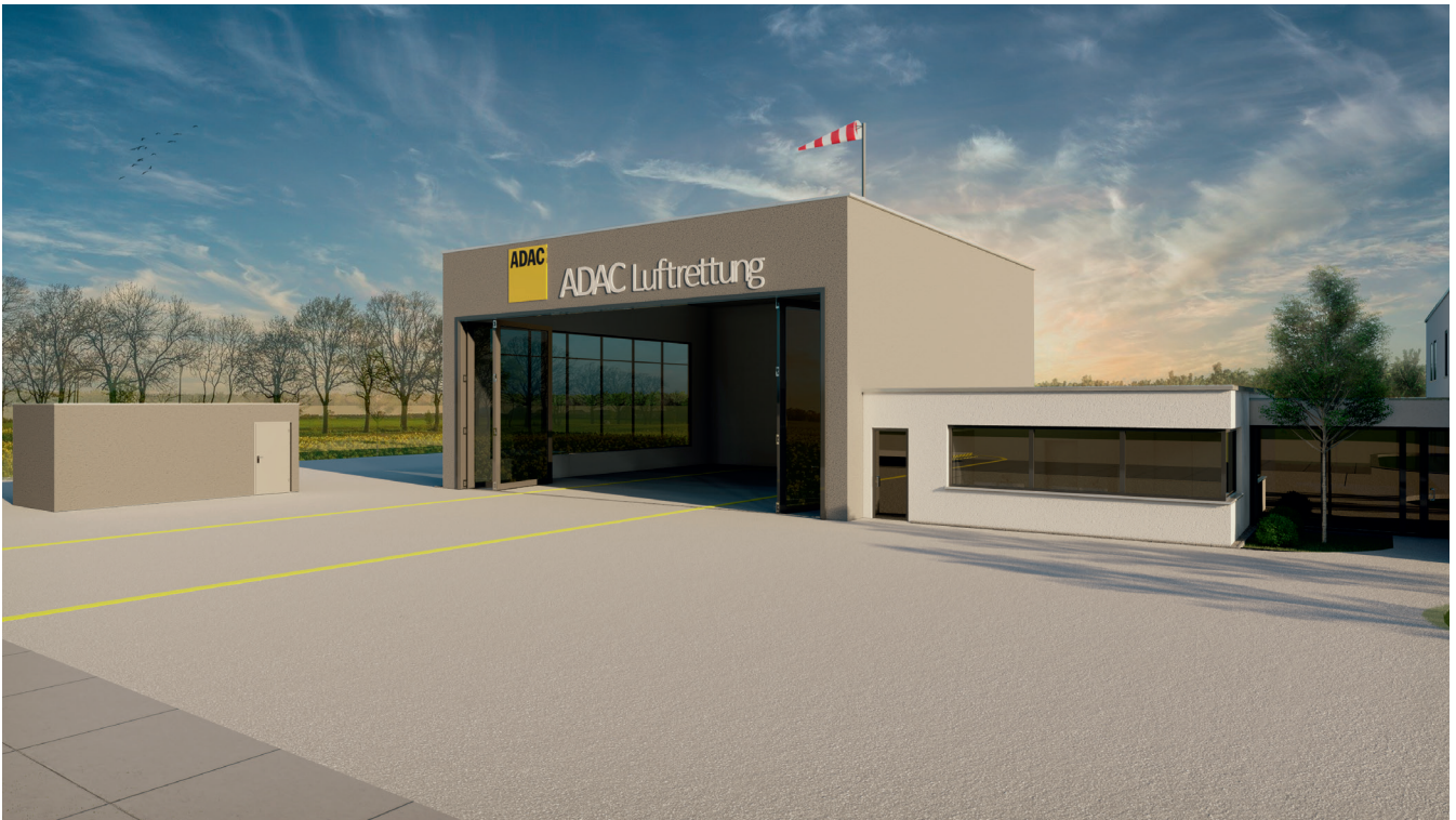
Figure 5.10: Example of a multicopter station as an extension of existing structures (Front view/detailed view)
